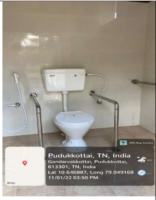
Divyangjan Toilet view II
