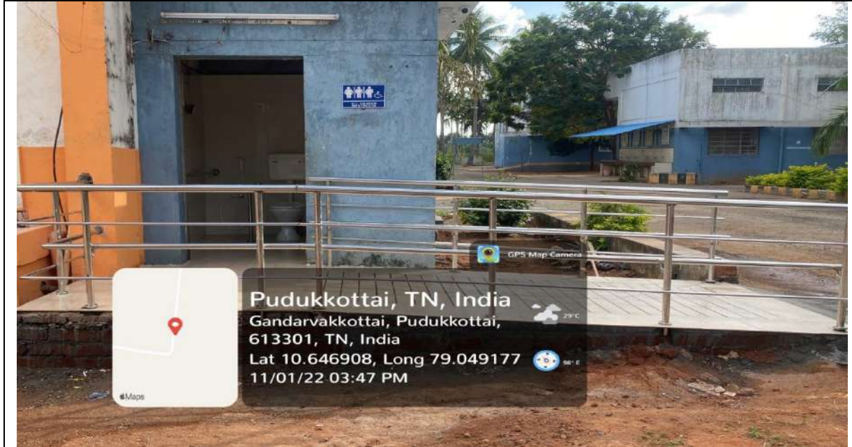
Divyangjan Toilet view V
